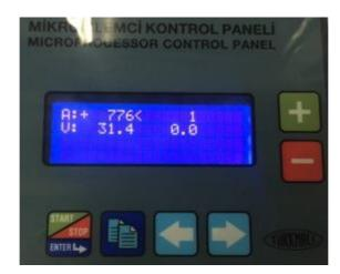
(A) (V) and current figures is the multiplier in front of volts. In this section, the transaction flow in rectifier panel of the rectifier output current or volts and volt reading is performed in the same manner. Do not forget to save your transactions with the ENTER key.
